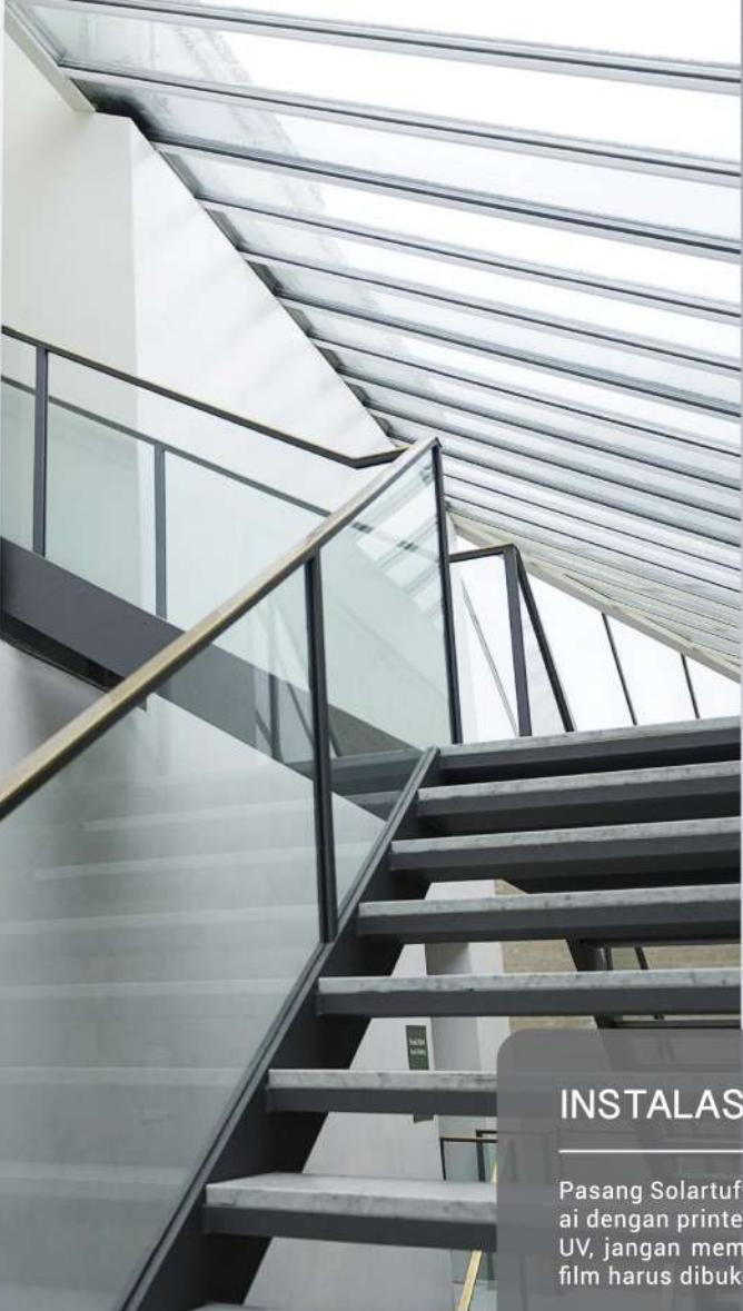
Always install UV protected side facing the sun (marked by printed masking). Before installation, do not remove the masking as it is not possible to determine the UV protected side once the film is removed. Masking should be removed maximum 2 days after the installation.
